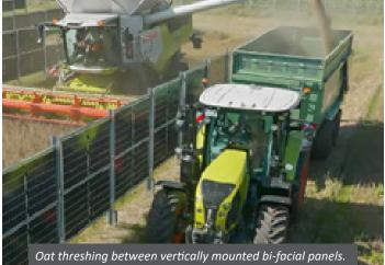
Vertical bifacial panels have photovoltaic cells on both sides of the panel and are installed facing east and west. They can generate electricity on the east facing side in the morning, and the west face in the afternoon. The vertical orientation allows for greater row spacing and flexible agricultural use simultaneously. Credit – Next2Sun
